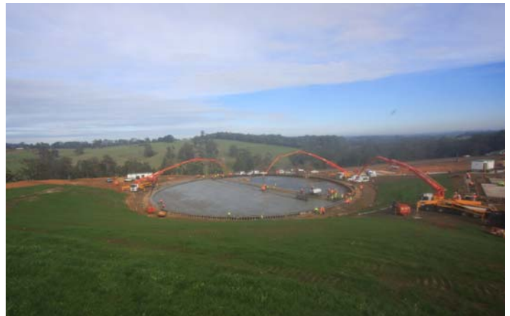
Treated water storage tank concrete pour
