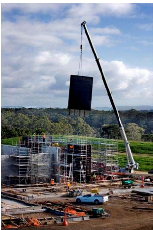
Main water treatment building
